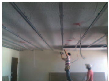
Living Room - false ceiling being installed
