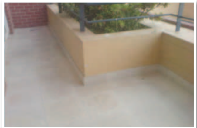
Balcony - After Renovation
