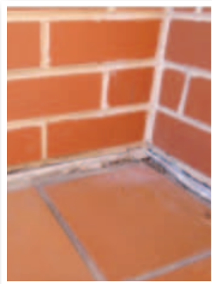
Balcony Close-Up - Before
