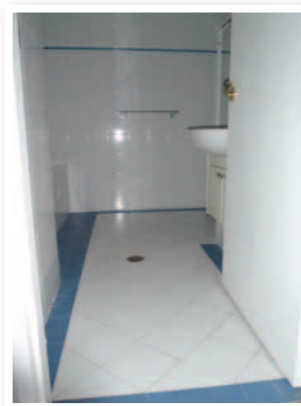
Main Bathroom - Before
