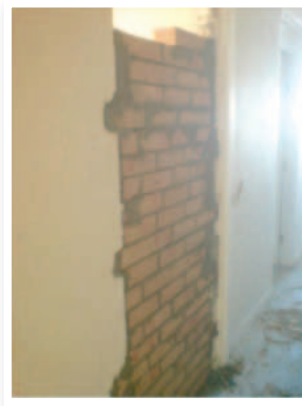
Separate Toilet - During
