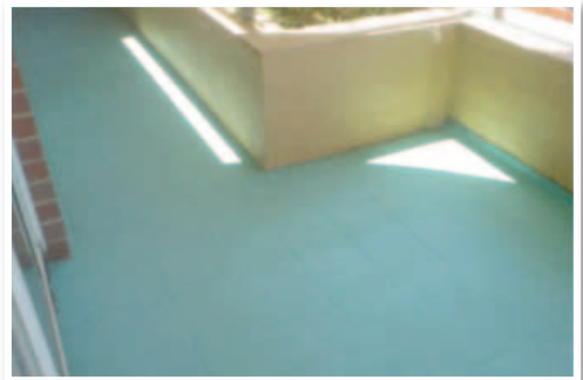
Balcony - During Renovation
