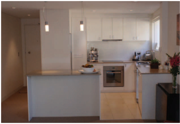
Wall removed and new kitchen installed
